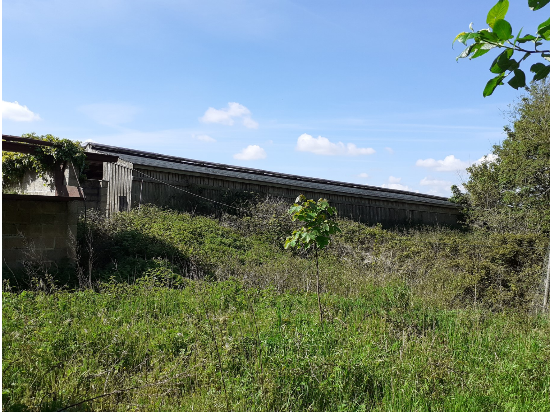
North (rear) elevation of Building C
