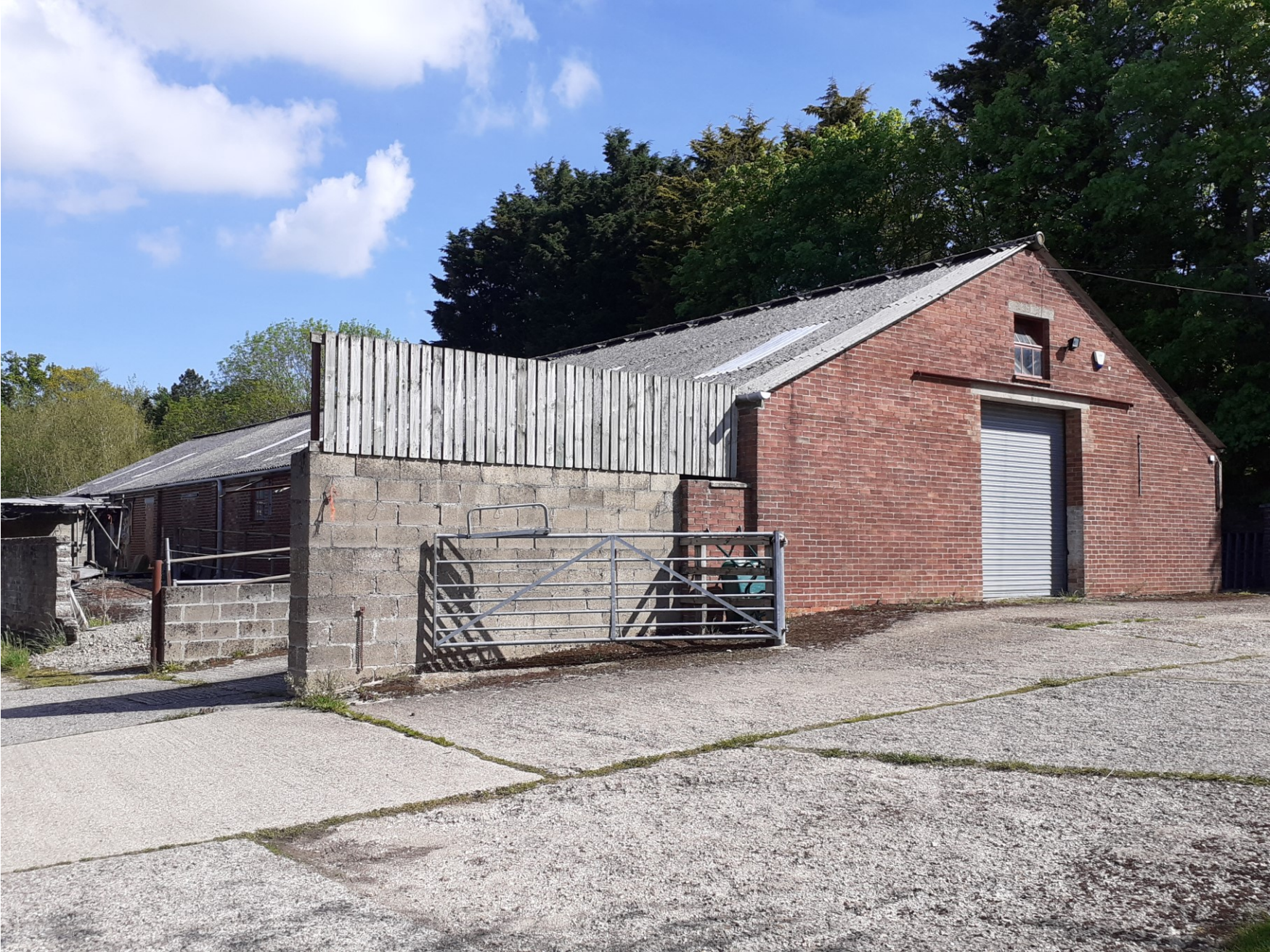
South elevation of Building A
