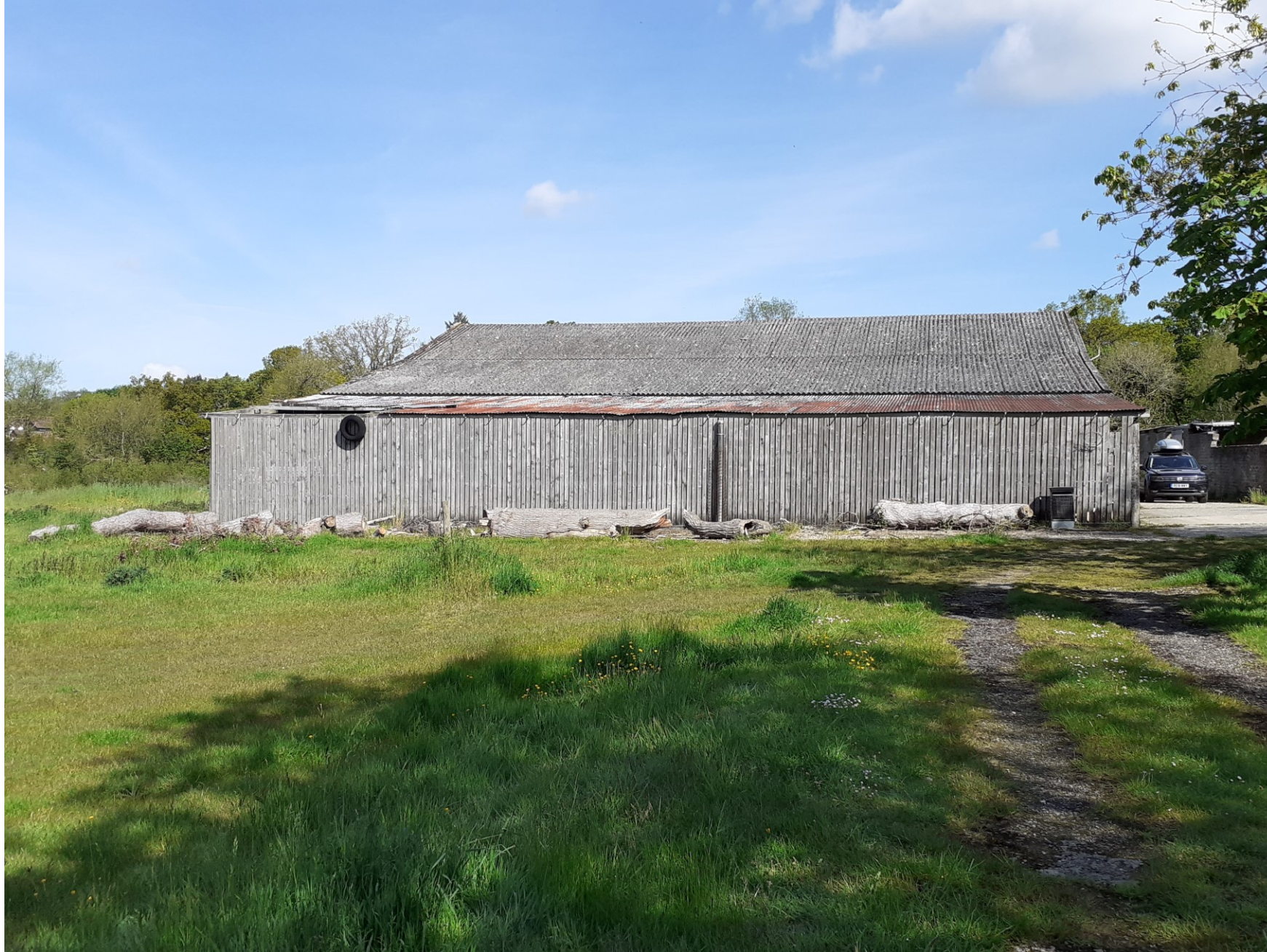
View of Building B (to be demolished) from the south
