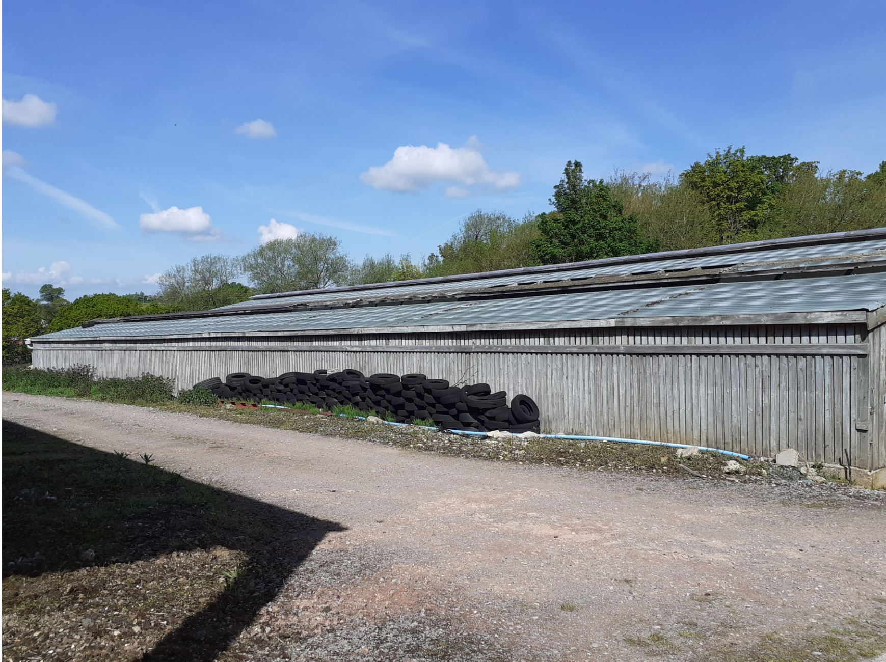
South (front) elevation of Building C
