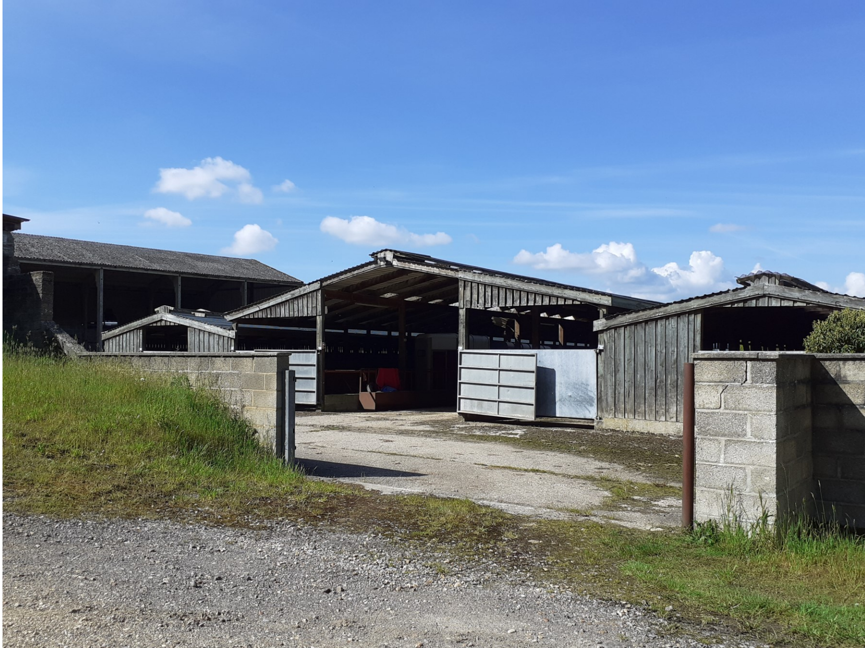
Side (east) elevation of Building C
