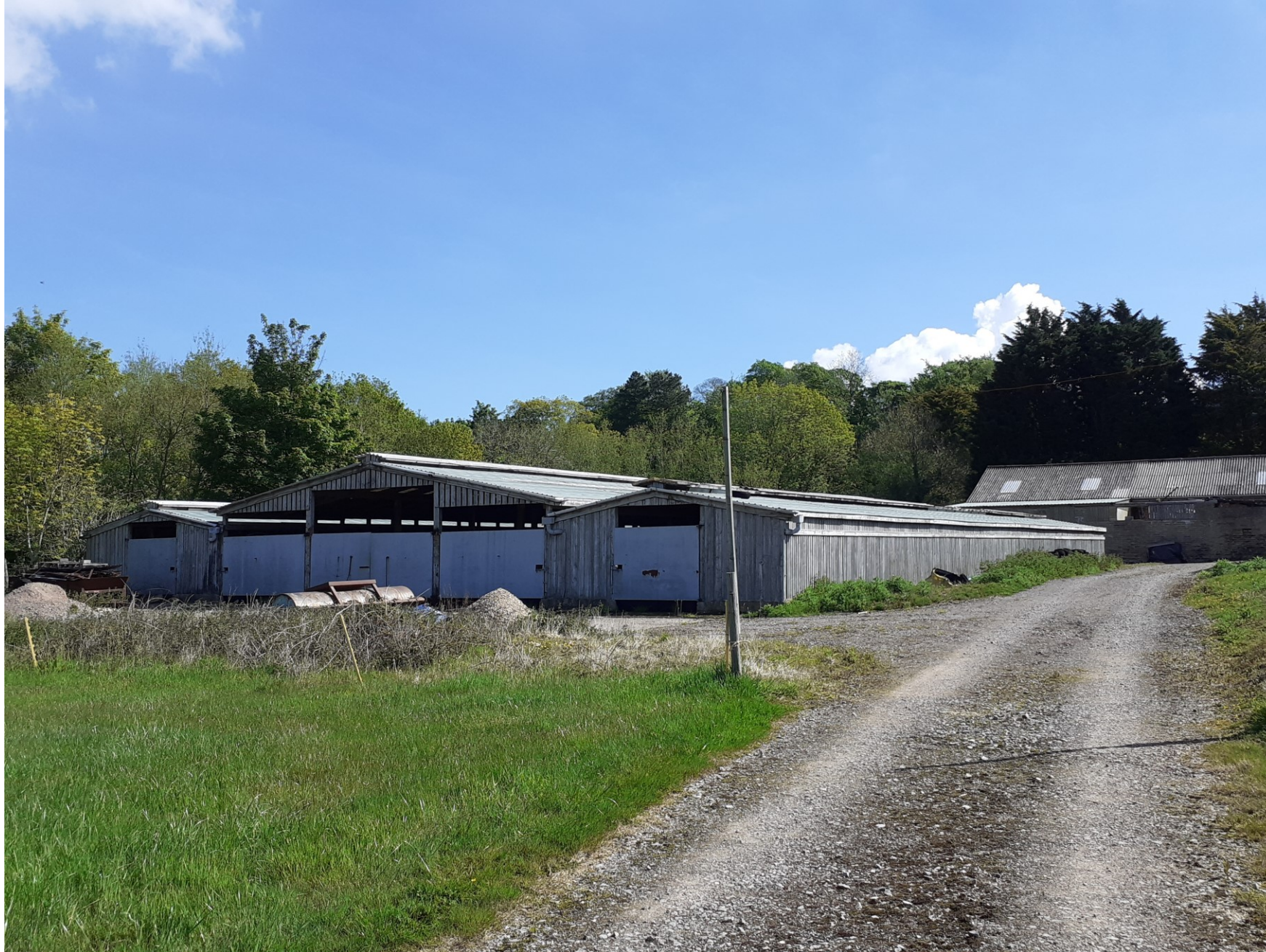
Building C (west and south) elevations viewed from access track
