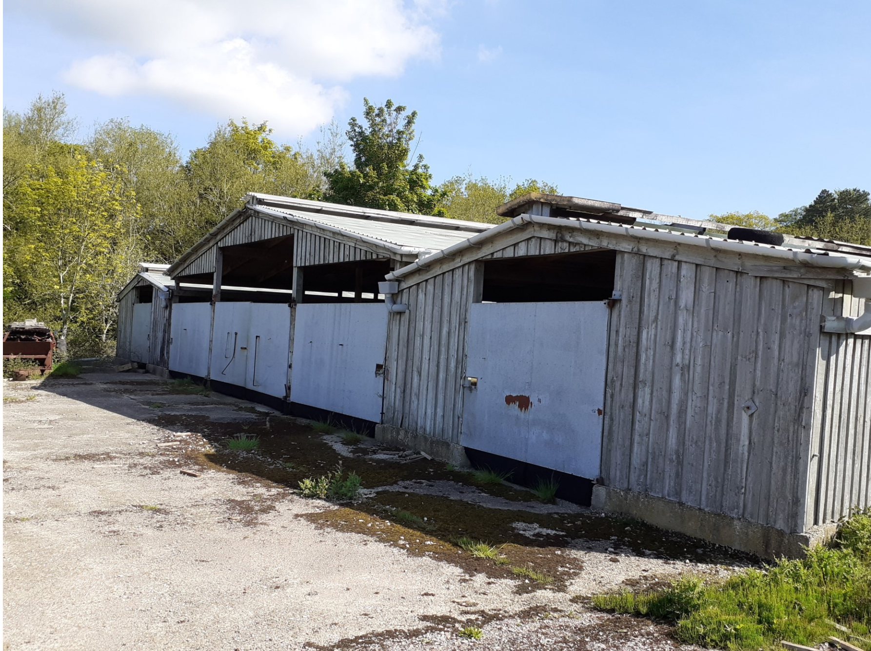
Side (west) elevation Building C
